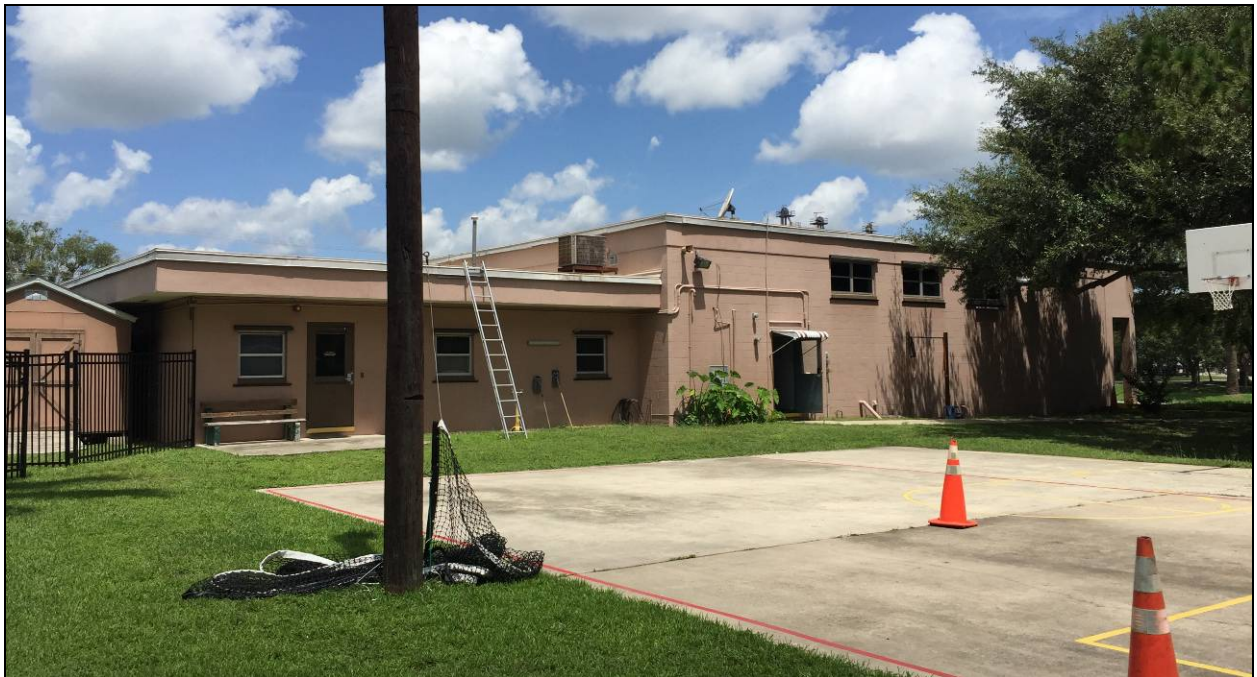
View of the east elevation of the fire station building from the east boundary of the site facing NWLY.
