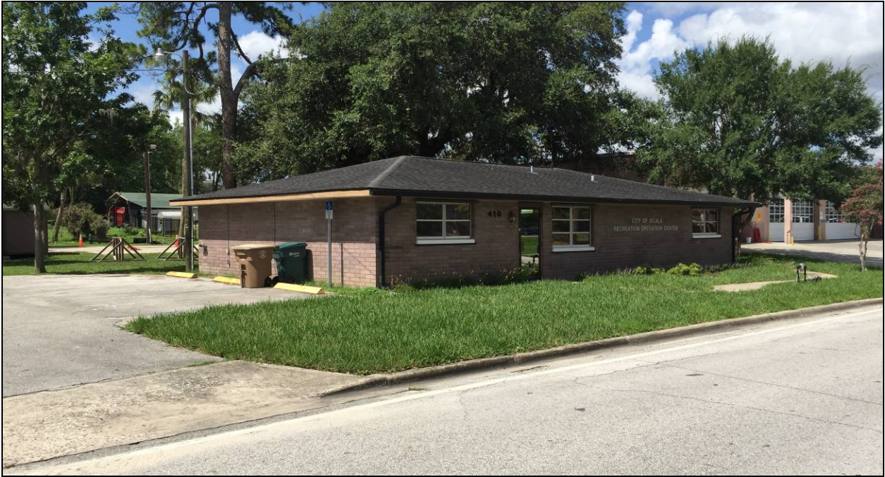
View of the former administrative building that is now being used by the Rec. Dept. It is planned for demolition.
